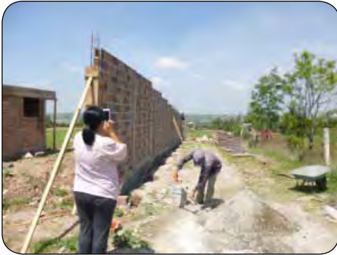
Volunteers raise the walls and roof of their new no-kill animal shelter.
